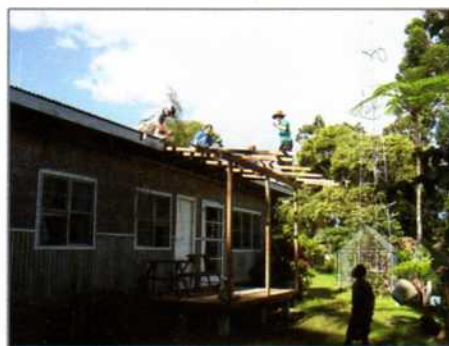
Building a porch on the Lutz's house
